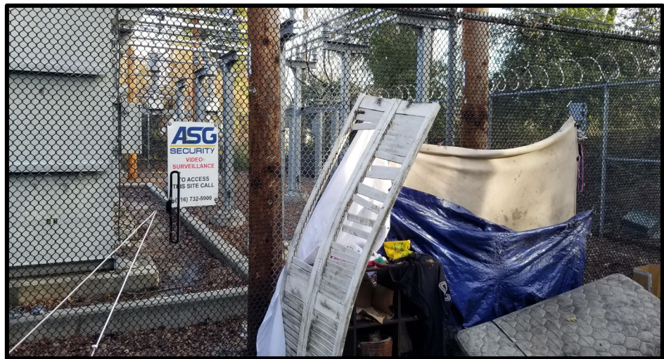
Figure 2 - SMUD Substation Encampment
