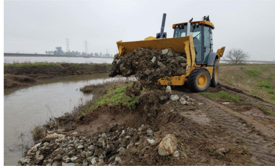
Repairing a slip in the levee in the Pleasant Grove area
