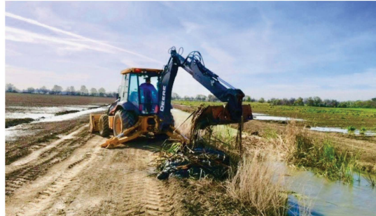
Silt removal from some of the interior drainage ditches
