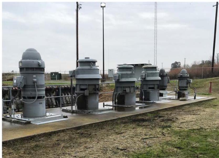
Figure 6 - Pumping Plant 3 Pumps
