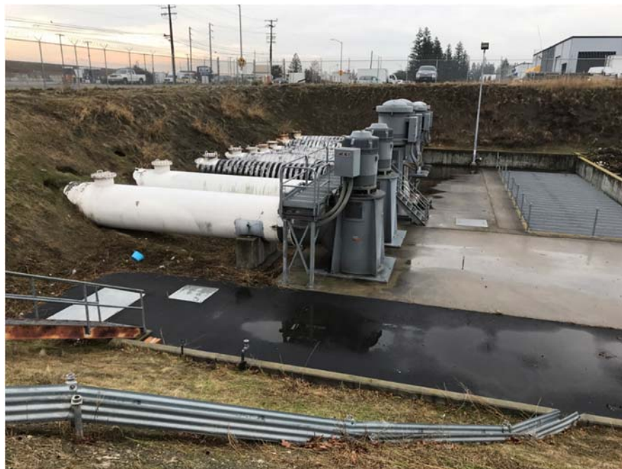
Figure 7 - Pumping Plant 8 Pumps
