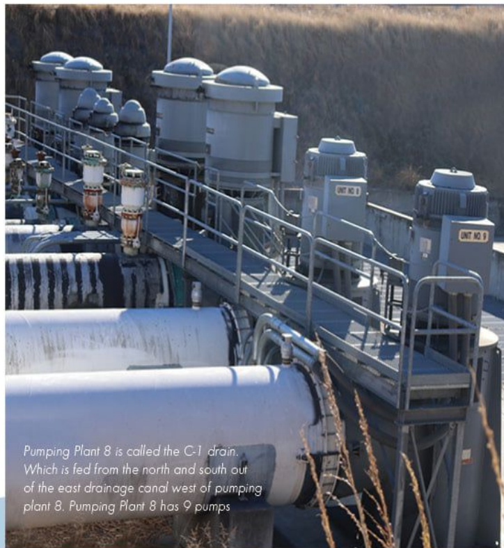
Army Corps Engineers Reach H project. The Corps replaced District 1000’s discharge pipes from Northgate Boulevard to Steelhead Creek.
